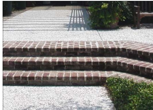
Aggregate Concrete with Brick Stairs
