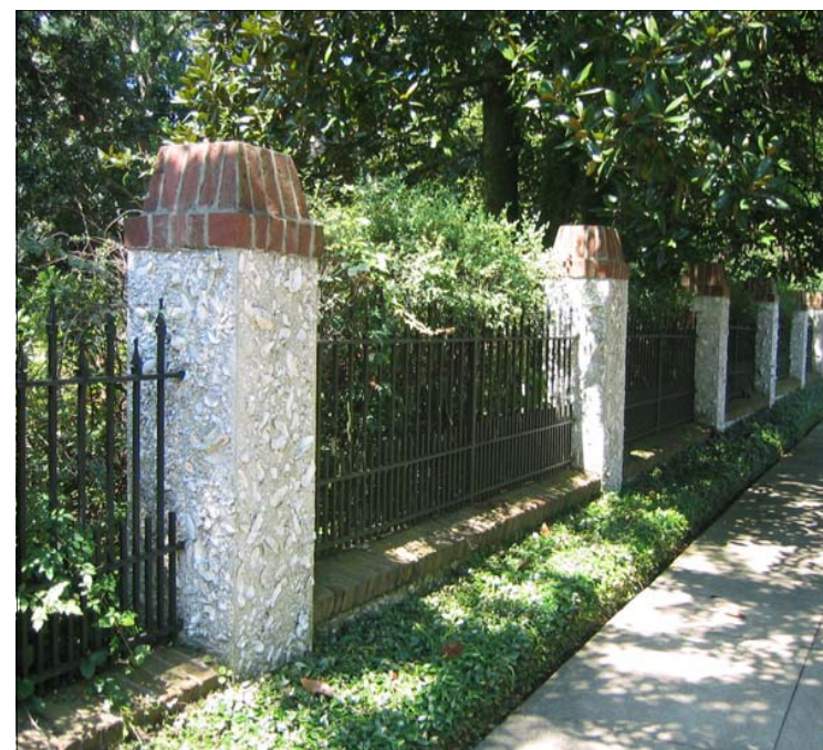
Wrought Iron Fence with Tabby Pillars
