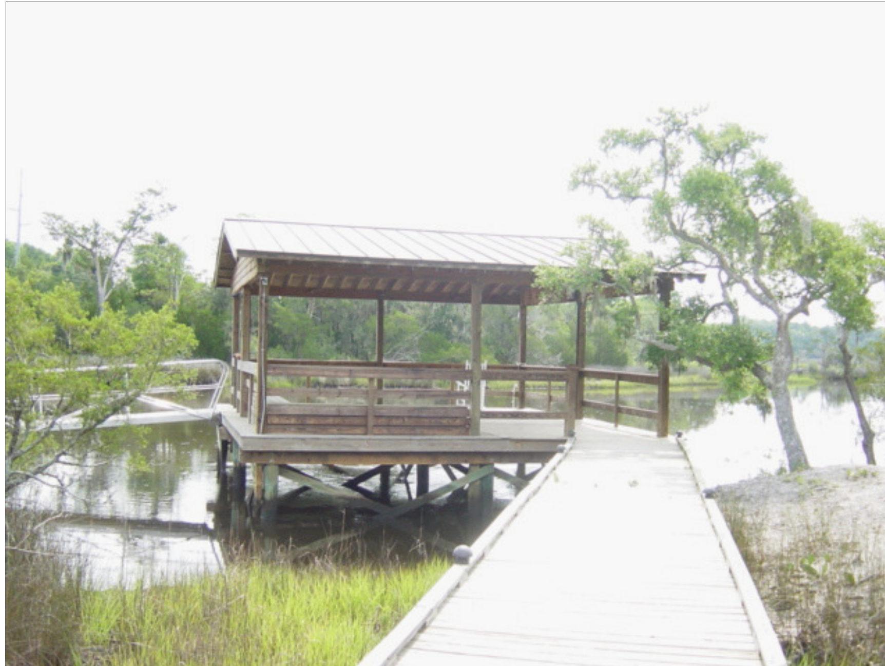
Poplar Grove Boathouse Community Dock
