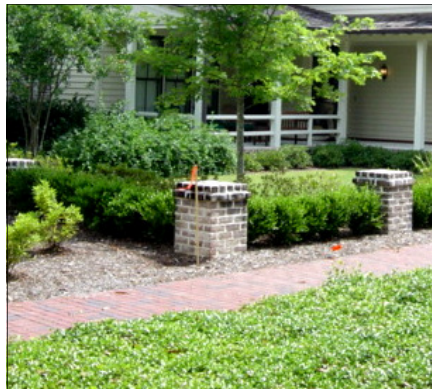
Hedge Fencing with Brick Pilasters
