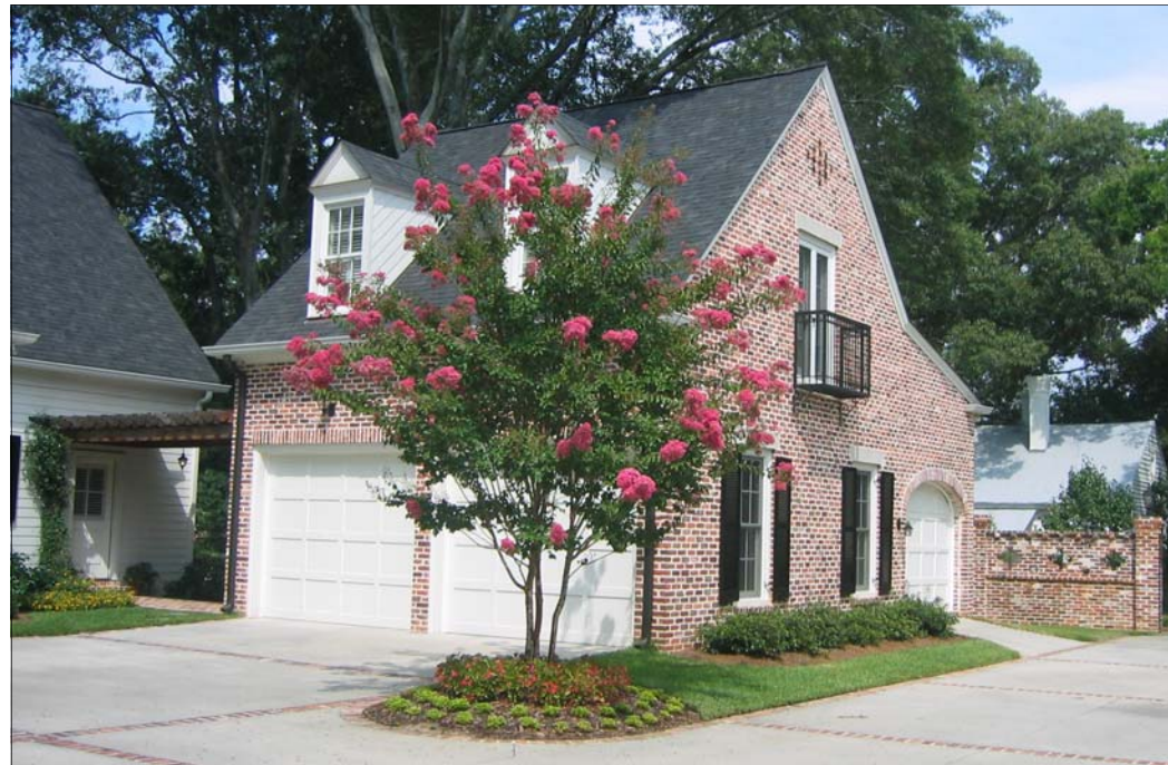
Double Doors with Dormers, Additional Side Door, and Living Quarters Above
