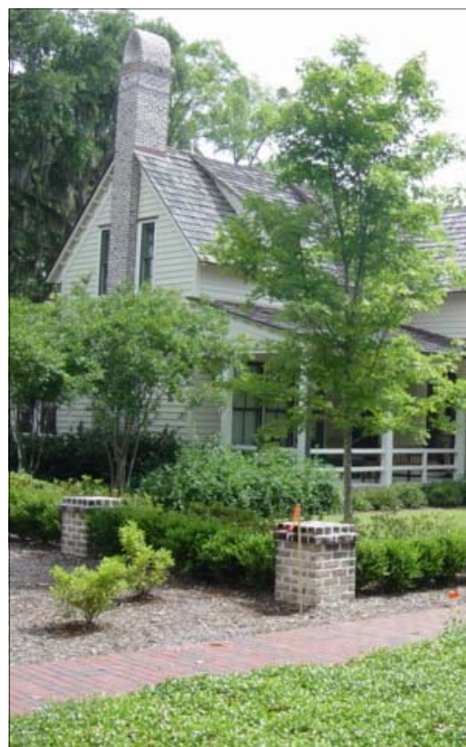
Brick Chimney and Foundation
