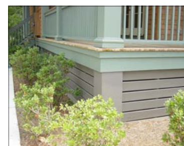
Stucco and Horizontal Fencing
