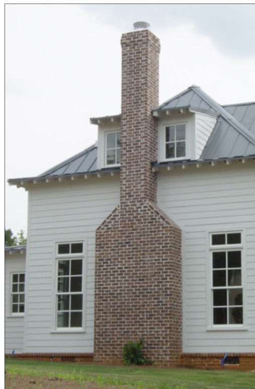
Brick Foundation and Chimney
