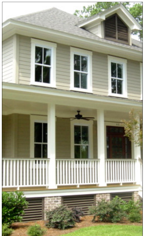
Windows without Shutters
