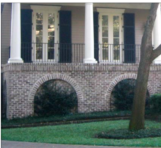
Brick Foundation with Arched Detail
