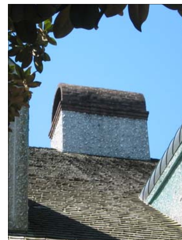
Tabby and Brick Chimney
