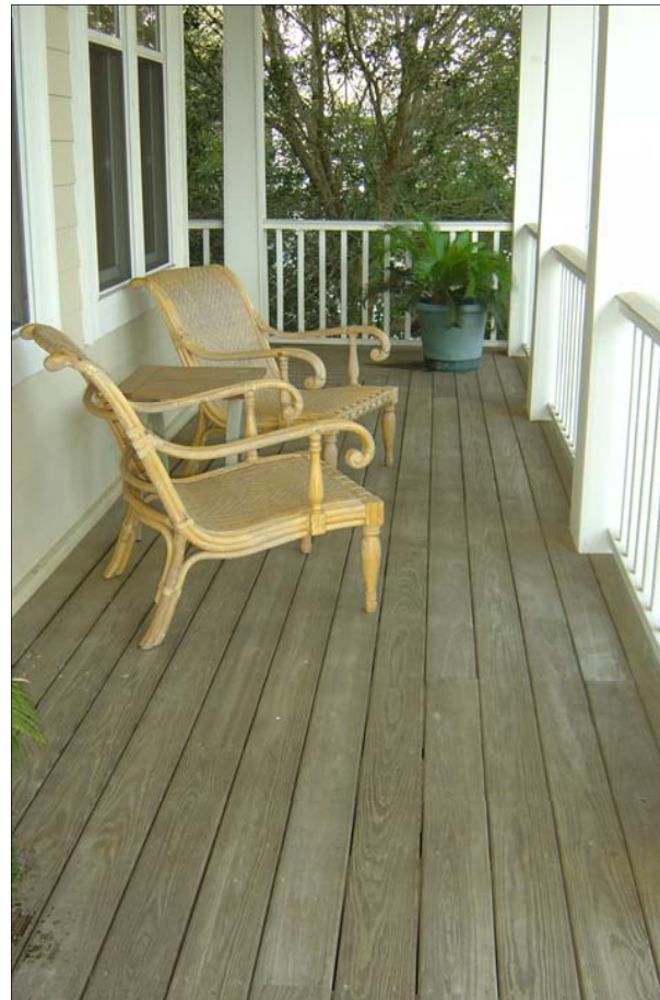
Treated Wood Floor (note: shallow porch discouraged)
