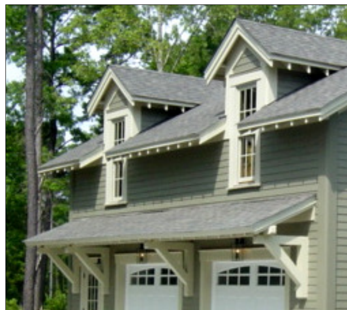
Exposed Rafter Tails with Bracketed Overhang
