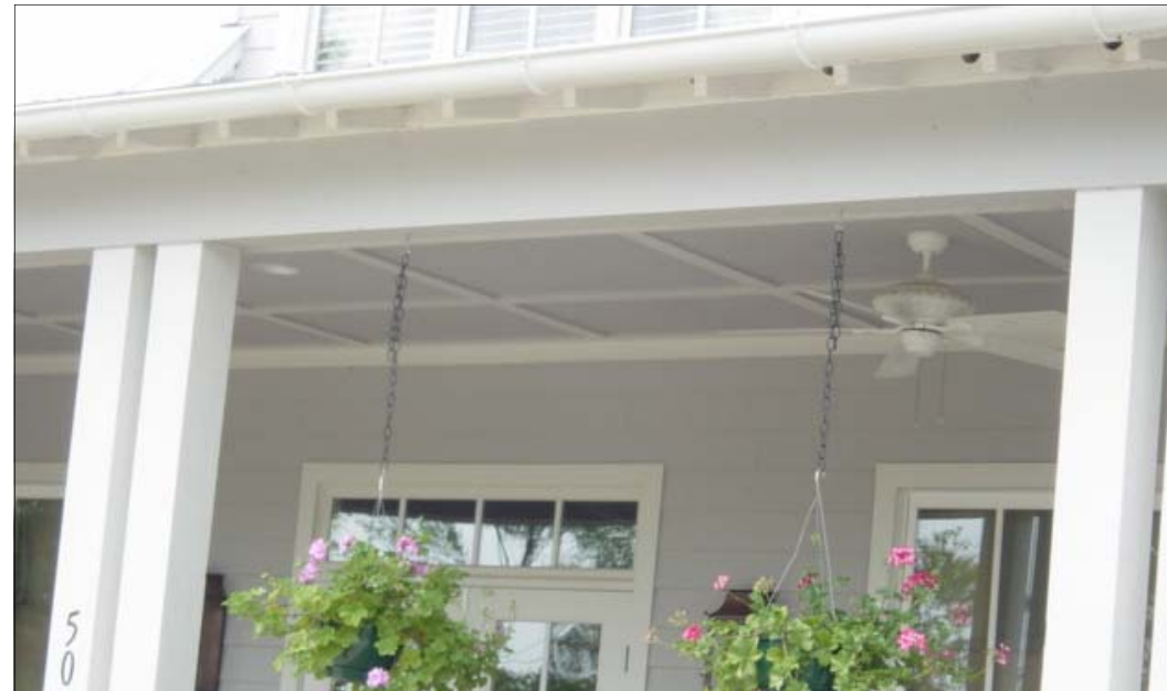
Painted Paneled Ceiling with Fans, Can Lights, and Exposed Rafter Tails
