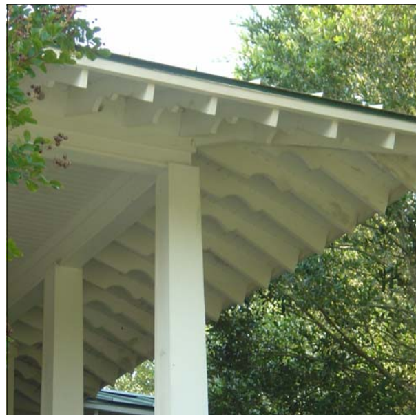
Bead Board Ceiling with Exposed Rafter Tails
