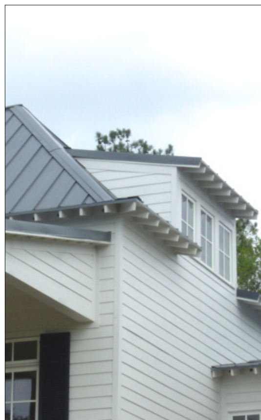
Exposed Rafter Tails
