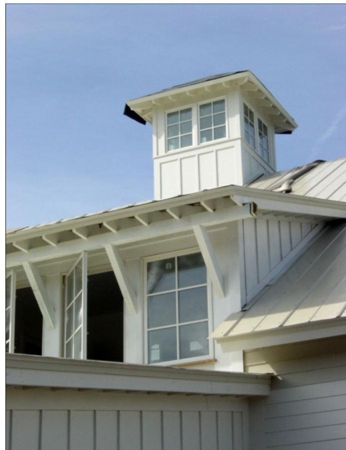
Exposed Rafter Tails with Bracketed Cornice
