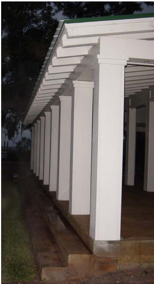
Square Doric Columns
