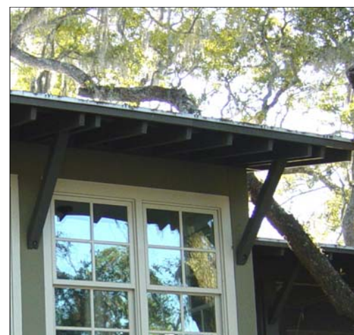
Exposed Rafter Tails with Bracketed Cornice
