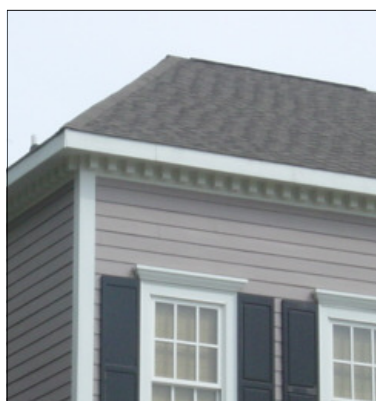
Cornice with Dental Molding
