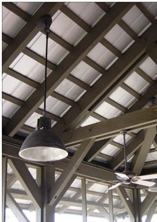
Exposed Metal Roof
