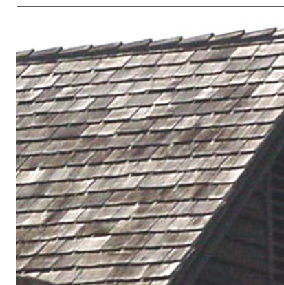
Shake or Shingle Roof
