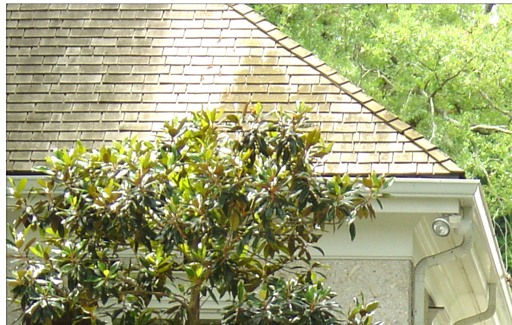
Shake or Shingle Roof
