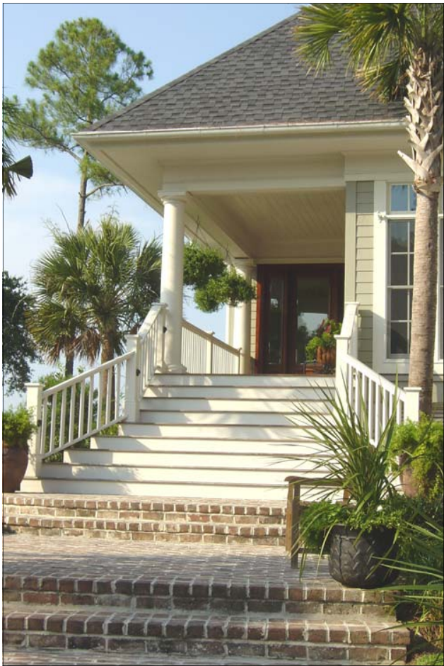
Angled Stair Rail
