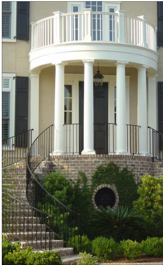
Curved Stair Wrought Iron Railing
