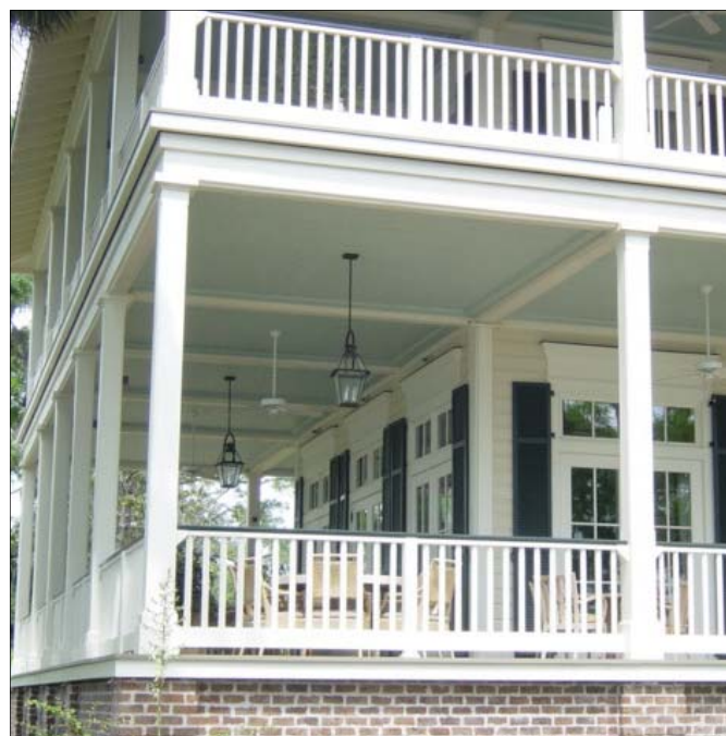
Two-Story Wrapping Porch
