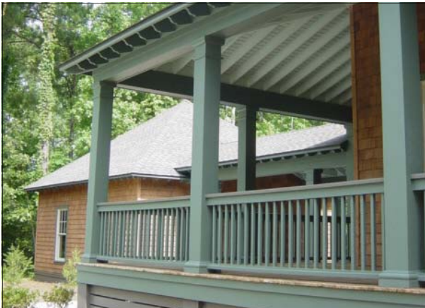
Square Doric Columns
