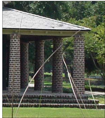
Round Tapered Brick Columns
