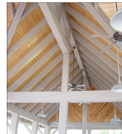
Exposed Roof Framing
