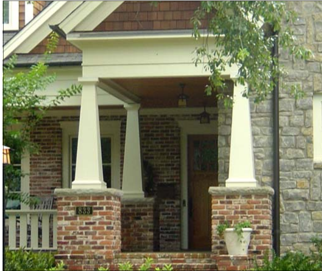
Square Tapered Columns on Piers
