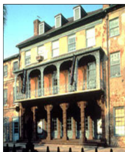
Dock Street Theater
