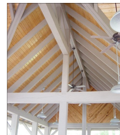
Exposed Roof Framing
