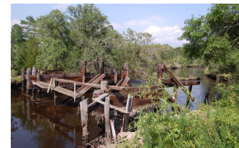
Remains of a dam gate used to maintain desired water levels
