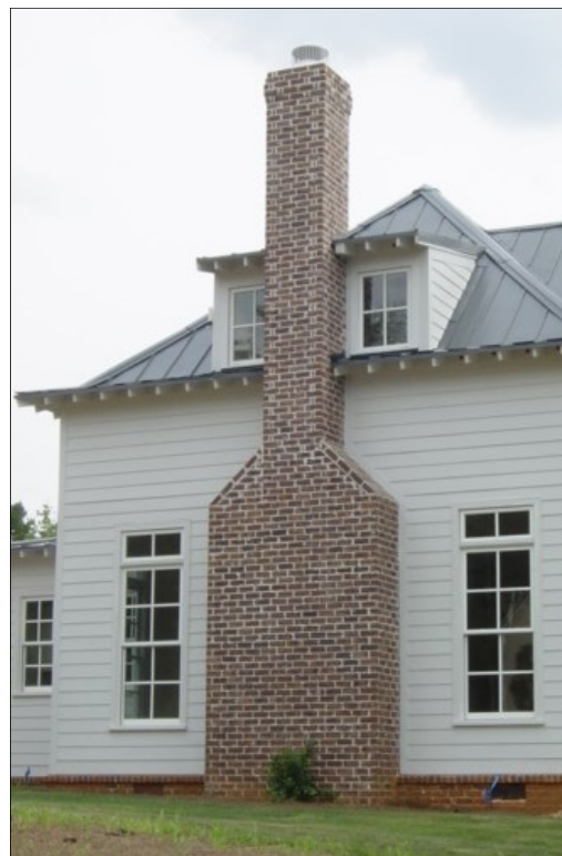
Brick Foundation and Chimney
