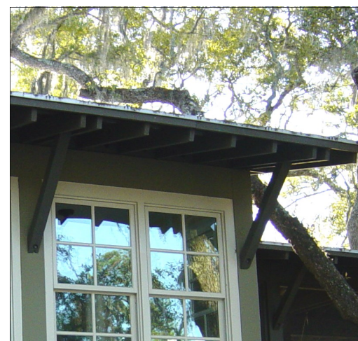
Exposed Rafter Tails with Bracketed Cornice
