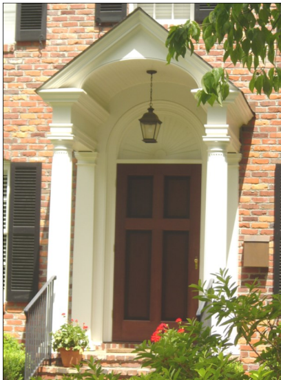
Pilasters and Engaged Columns
