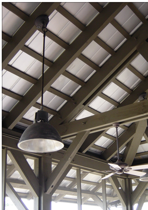
Exposed Metal Roof
