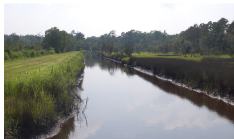
Flood canals wind throughout Poplar Grove
