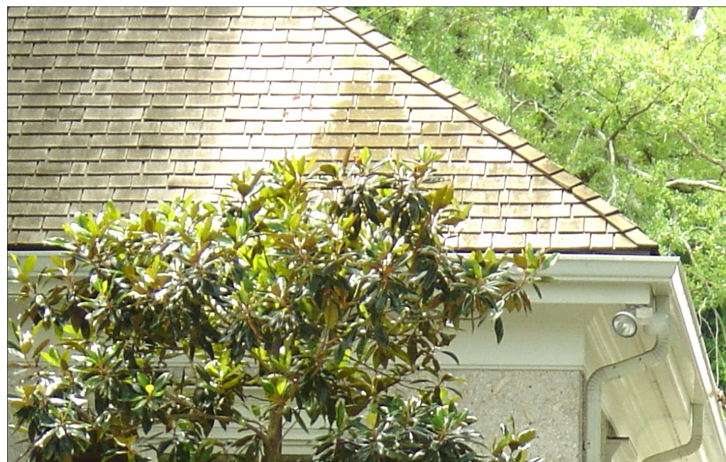
Shake or Shingle Roof
