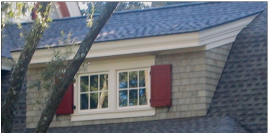
Shed Dormer with Double Window
