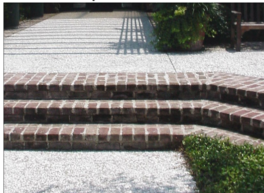
Aggregate Concrete with Brick Stairs
