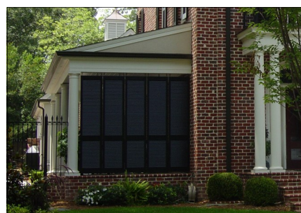
Side Porch with Louvered Shutters
