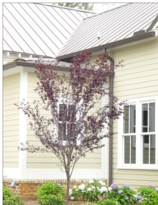
Hand-Crimped Standing Seam Roof
