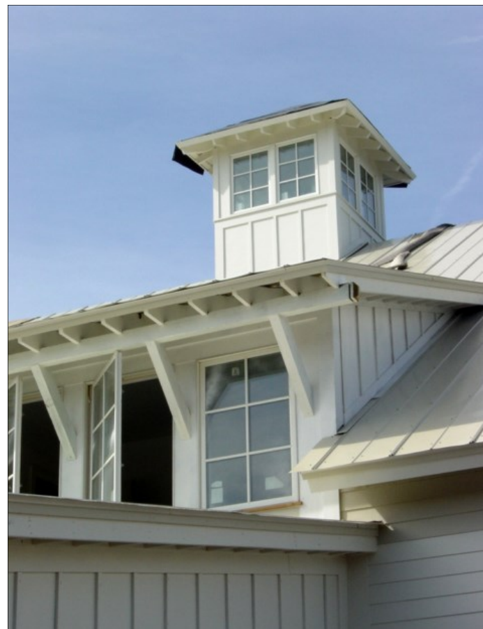
Exposed Rafter Tails with Bracketed Cornice
