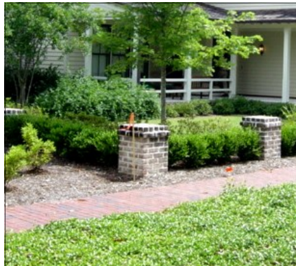
Hedge Fencing with Brick Pilasters
