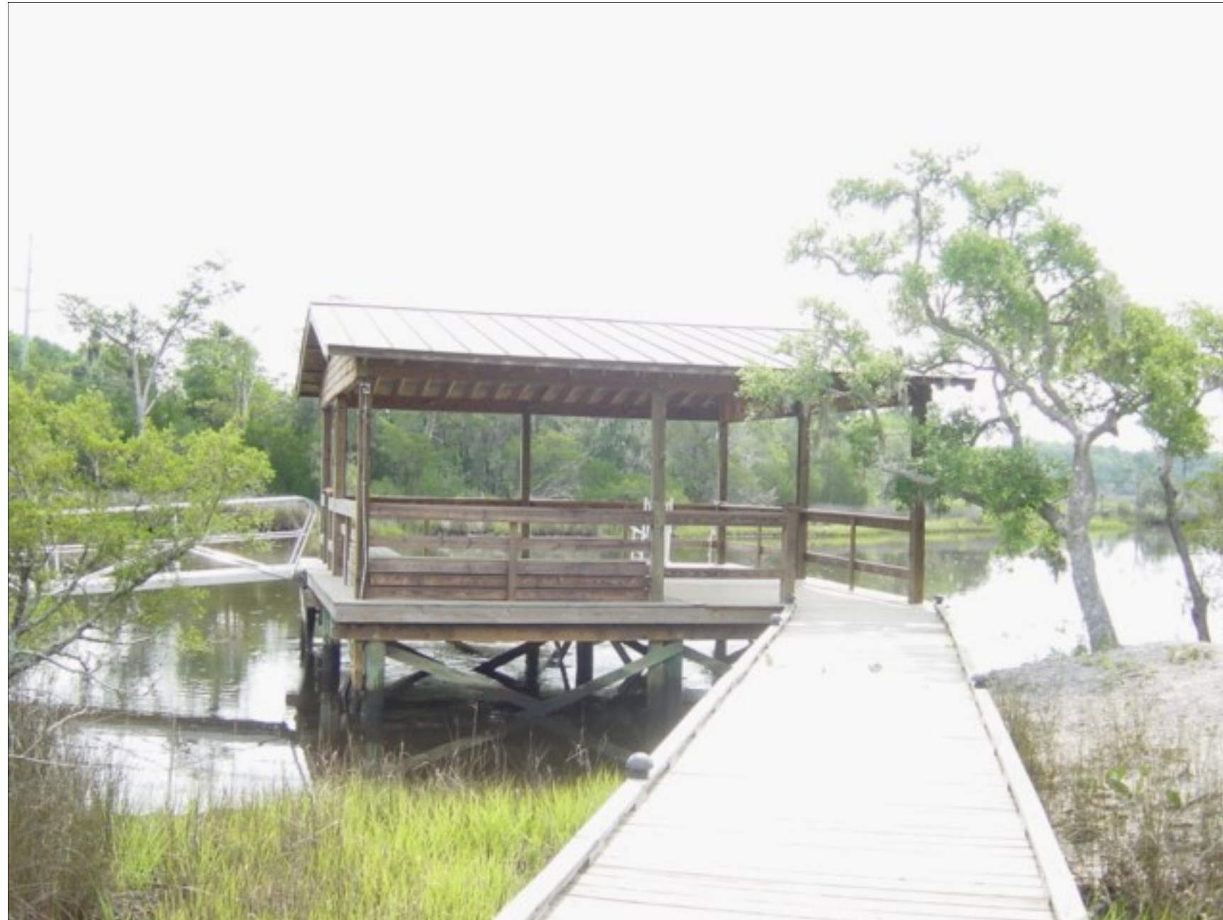
Poplar Grove Boathouse Community Dock
