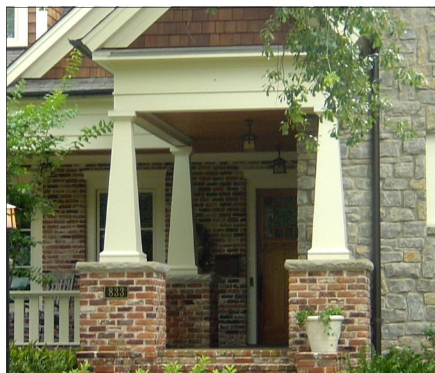
Square Tapered Columns on Piers
