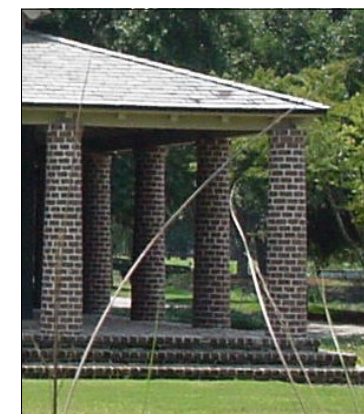
Round Tapered Brick Columns
