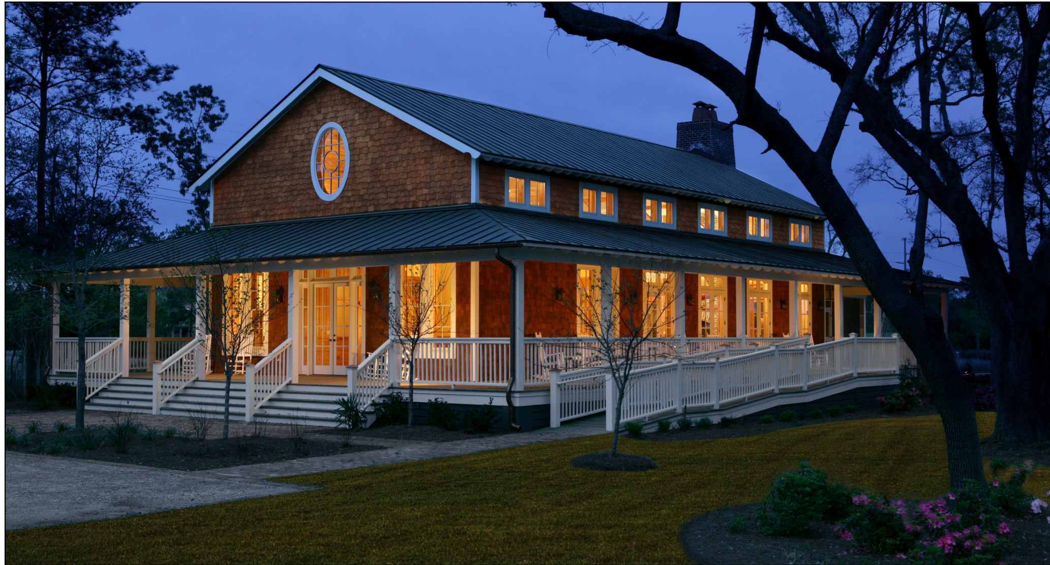
Poplar Grove Community Boathouse
