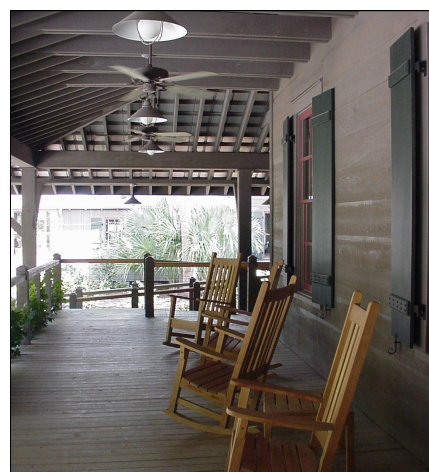
River Style Porch/Exposed Rafters
