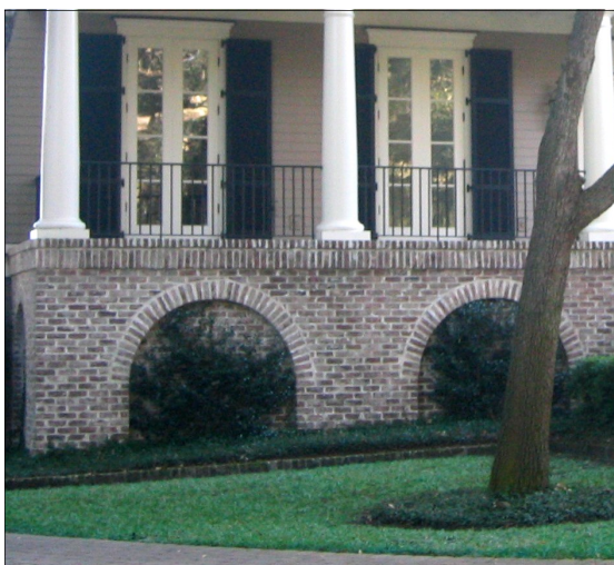
Brick Foundation with Arched Detail
