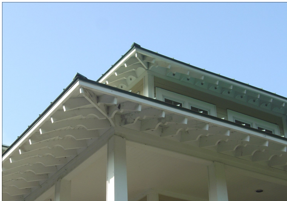
Exposed Cornice with Exposed Rafter Tails
