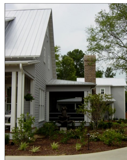
Side Screened Porch
