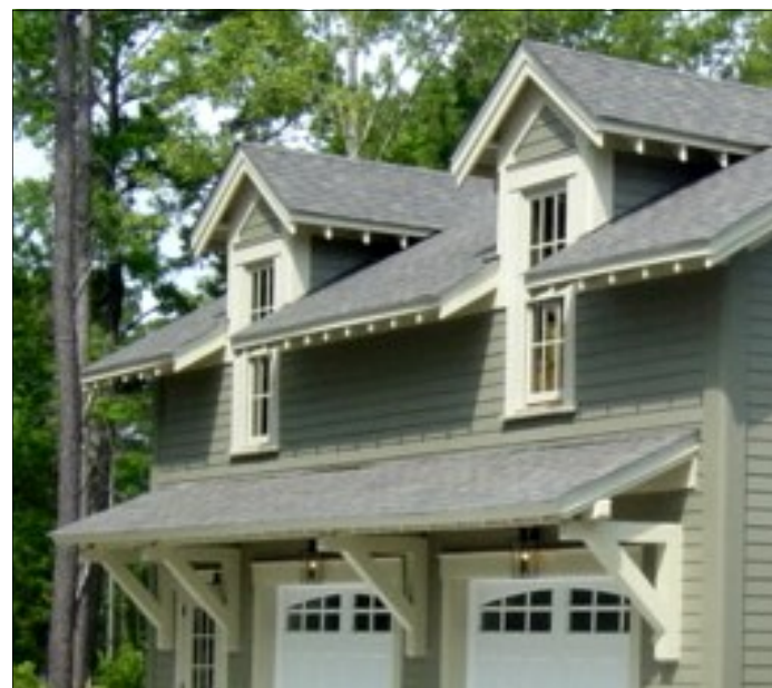
Exposed Rafter Tails
