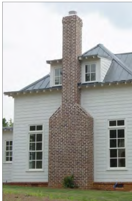
Brick Foundation and Chimney
