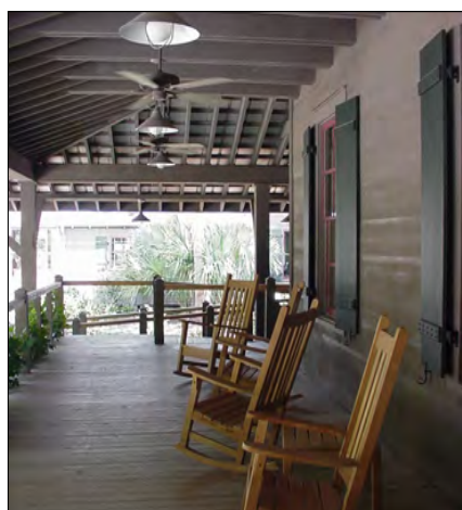
River Style Porch/Exposed Rafters
