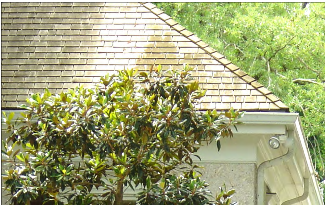
Shake or Shingle Roof
