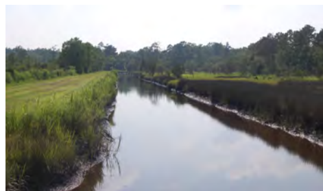
Flood canals wind throughout Poplar Grove
