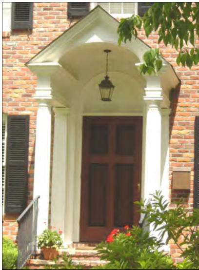
Pilasters and Engaged Columns
