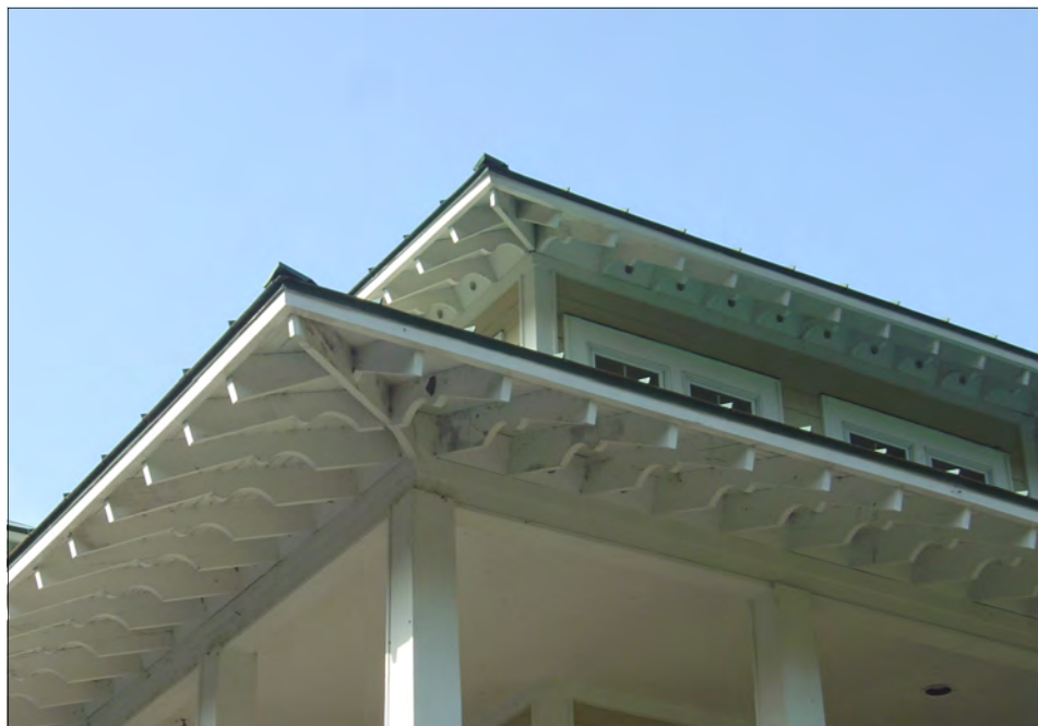
Exposed Cornice with Exposed Rafter Tails
