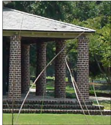
Round Tapered Brick Columns
