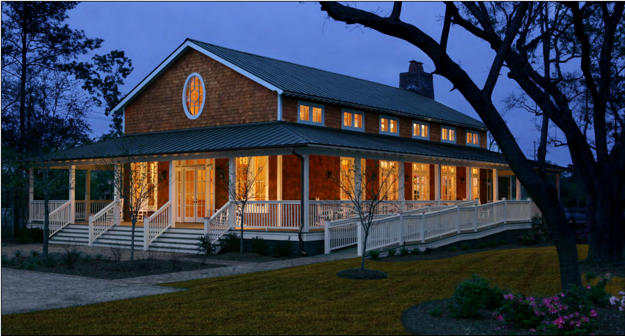
Poplar Grove Community Boathouse
