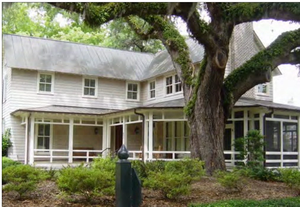
Single Story Wrapping Porch with Screened Section
