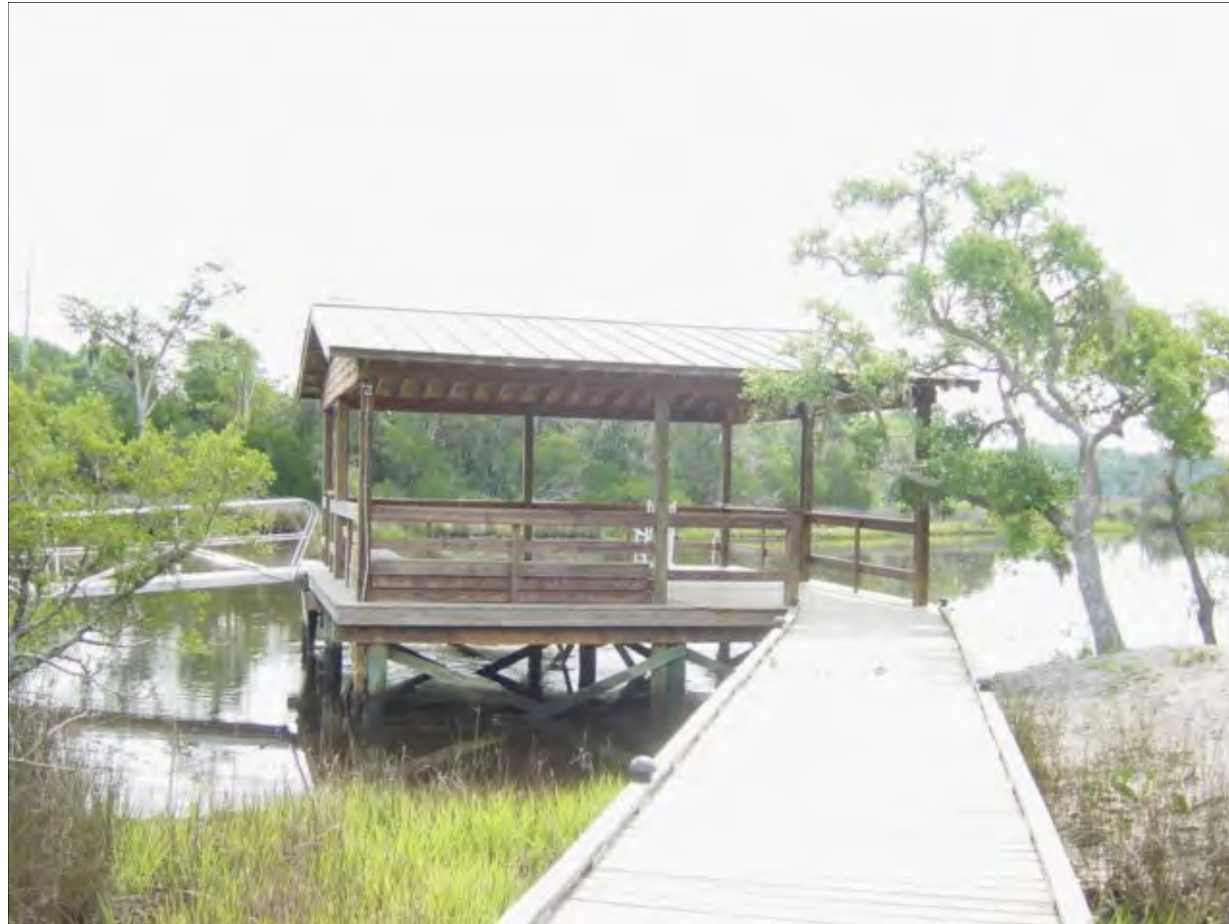
Poplar Grove Boathouse Community Dock
