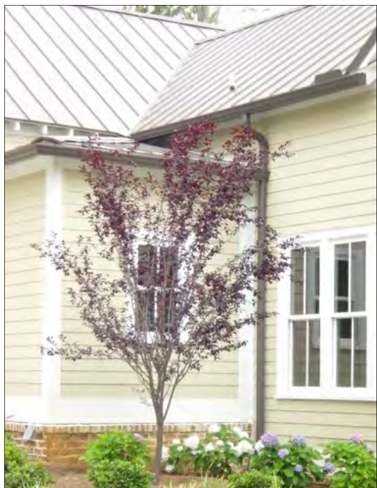
Hand-Crimped Standing Seam Roof
