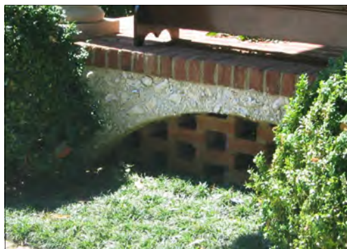
Tabby Foundation w/ Pierced Brick Detail
