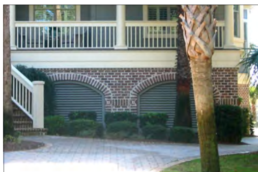
Brick Foundation w/ Arched Fencing Detail
