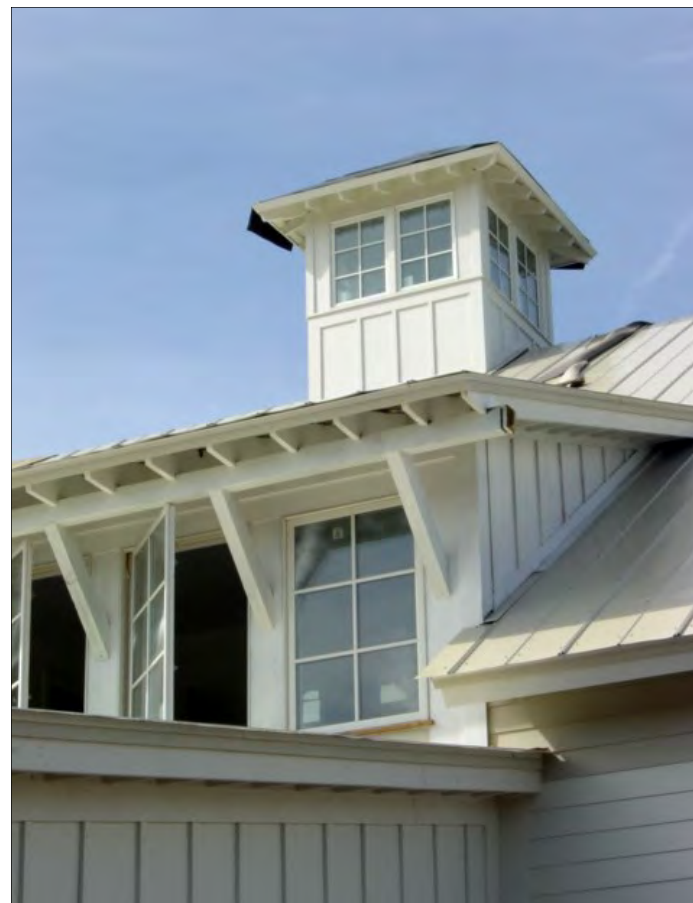
Exposed Rafter Tails with Bracketed Cornice
