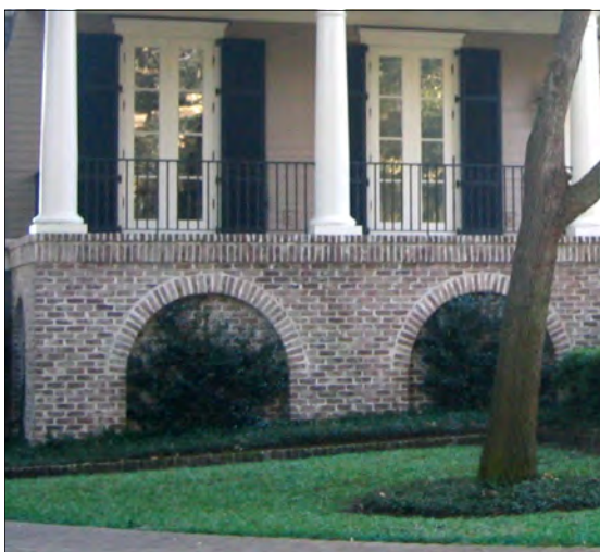
Brick Foundation with Arched Detail
