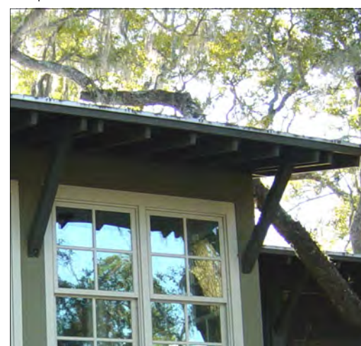
Exposed Rafter Tails with Bracketed Cornice
