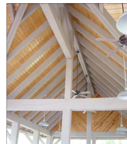
Exposed Roof Framing
