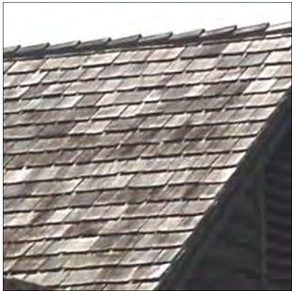
Shake or Shingle Roof
