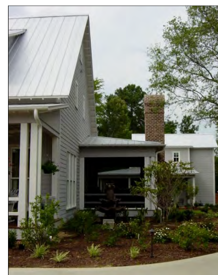
Side Screened Porch
