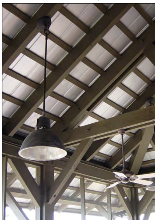
Exposed Metal Roof
